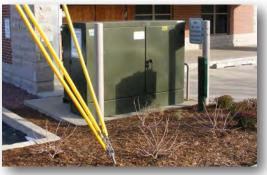
**Image 25:** The preferred location for a transformer is on a rear facade where adequate service access is provided.
