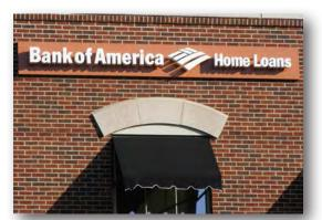
**Image 28:** Individual letters are applied to a panel to minimize damage to underlying masonry. Colors are complementary to the building.
