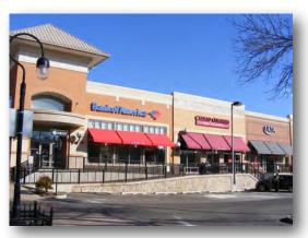
**Image 4:** Variations in the exterior wall plane subdivide the facade on this single building into multiple vertical storefront segments
