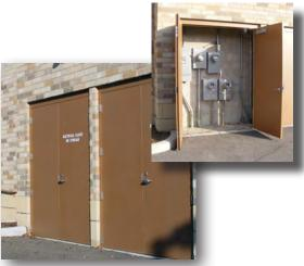
**Image 24**: Electric meters may be placed within an exterior closet (typically not greater than 18").
