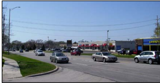
A. Between Ellsworth and Brainard Streets City of Naperville Electric (Removed during the course of the study)
