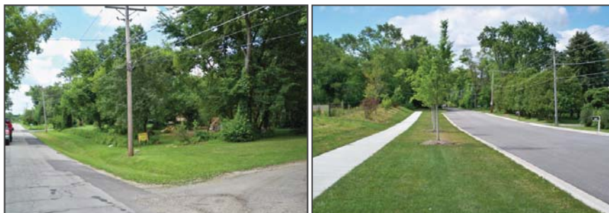
Pictured Left: Southern portions of Radcliff Road remain unimproved. Pictured Right: Northern portions of Radcliff Road have been improved as a result of teardown and infill development.
