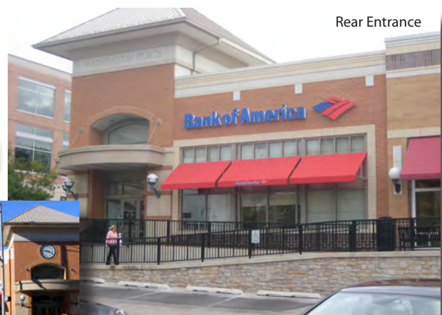
Rear Entrance at Washington Square Photos by City of Naperville
