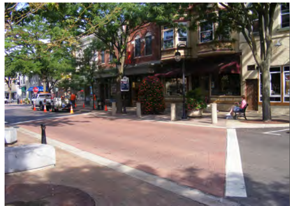
Jefferson Avenue Mid-Block Crossing Photo by City of Naperville
