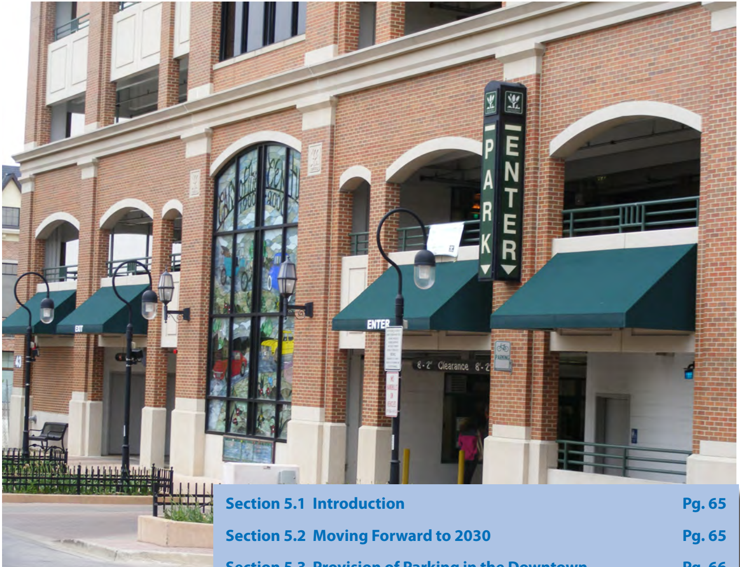
Van Buren Parking Deck Photo by City of Naperville
