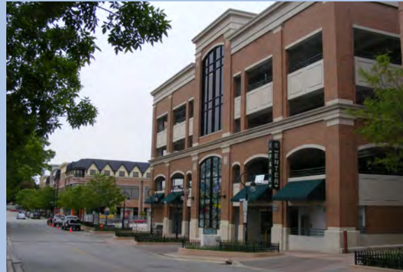
Van Buren Parking Deck Photo By City of Naperville
