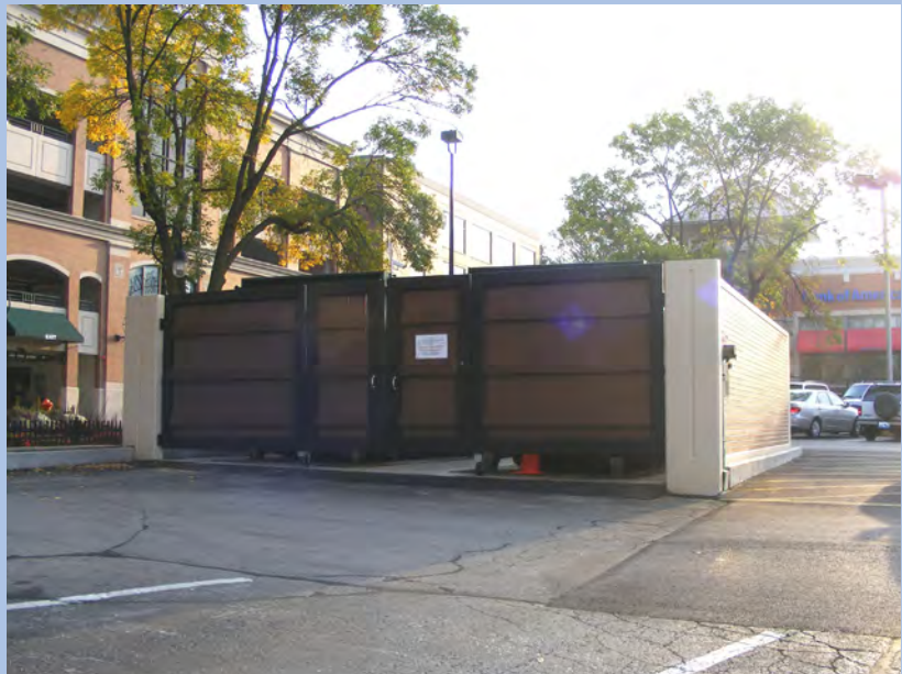
Van Buren Refuse Enclosure Photo by City of Naperville
