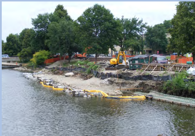
Riverwalk Construction between Eagle and Webster Streets Photo By City of Naperville
