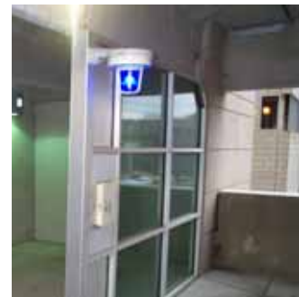
Picture 34: Emergency phone identified with blue light
