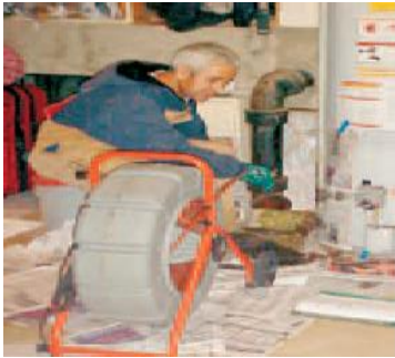
Locating the pipe
