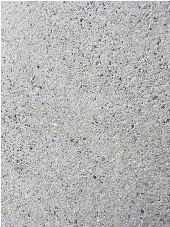
45. A close-up of the precast fin showing surface finish and exposed aggregate.
