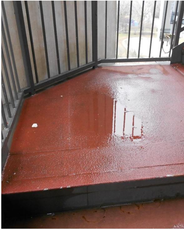
37. Standing water on stair landing.
