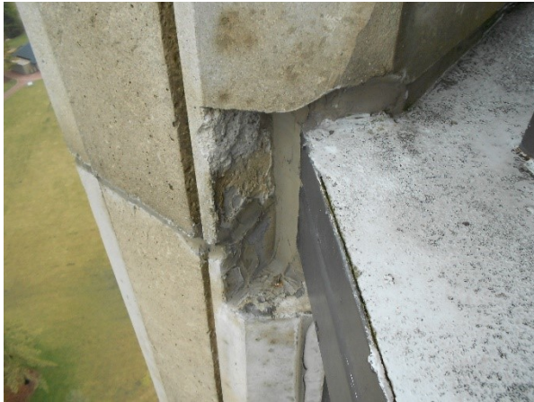
91. A close-up of open deck angle and traffic coating at the Observation deck level. .
