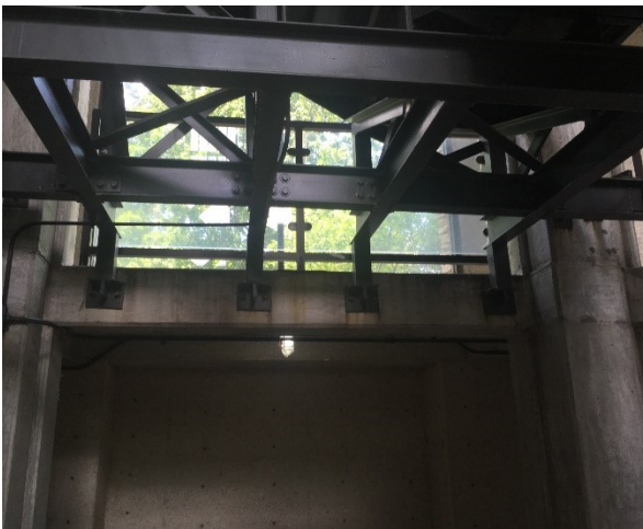
21. A view of the hanging stair structure from the basement. Note the 4 lateral braces.
