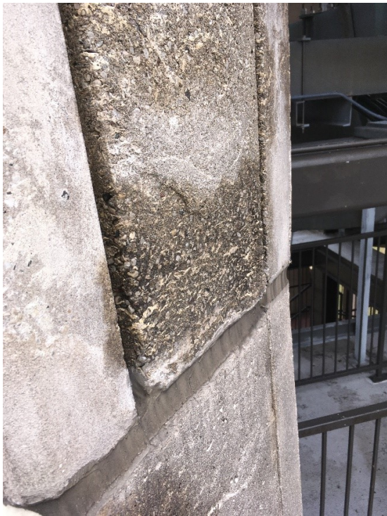
51. An example of surface discoloration from poor concrete consolidation.
