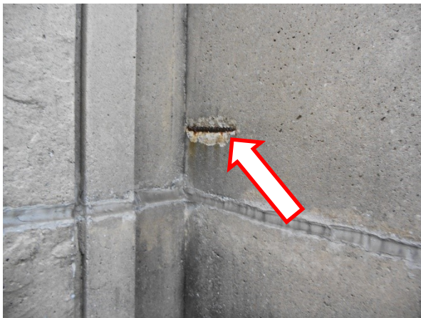
33. A close-up view of small rebar spalls
