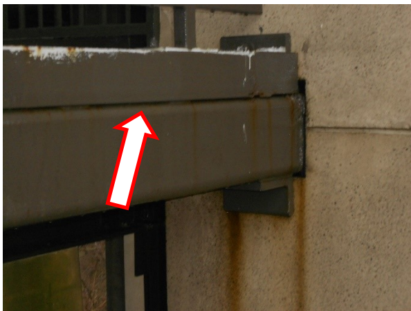
77. A view of typical corrosion at non-galvanized deck edge and ring beam. Note corrosion staining on precast fin.
