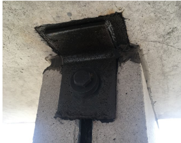
86. A close-up of fin connection in main piers.
