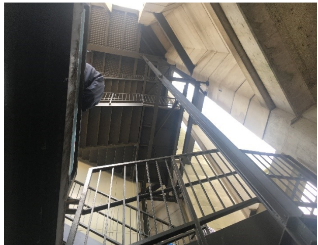
22. A view of the hanging stair structure from the ground level.
