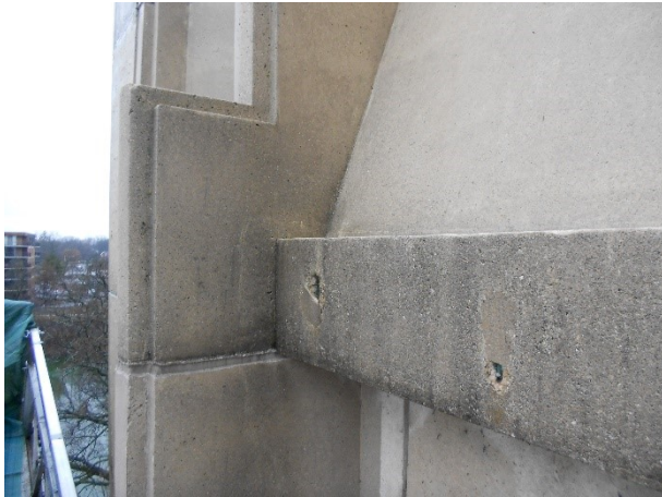
31. A close-up view of small rebar spalls
