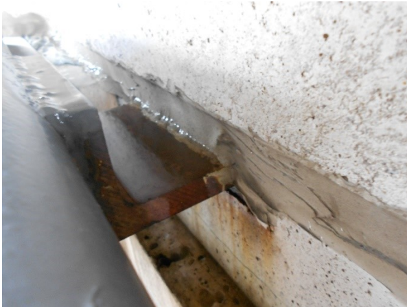
69. A close-up view of clip angle in precast concrete joint from above.
