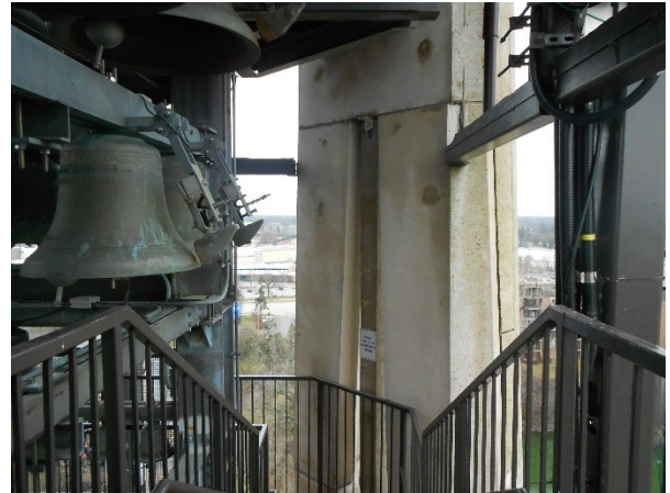
76. A view of horizontal carillon framing.
