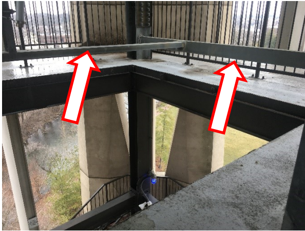
75. A view of horizontal carillon framing at the Belfry level.
