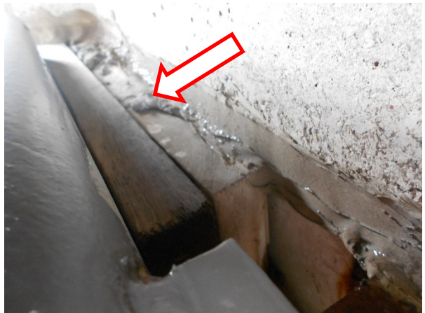
72. A close-up view of leftover wood blocking at ring beam connection.
