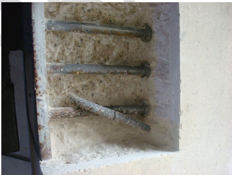
Photograph #7: Exposed connection plate and embedded studs at northwest side of Elev. 52.5.
