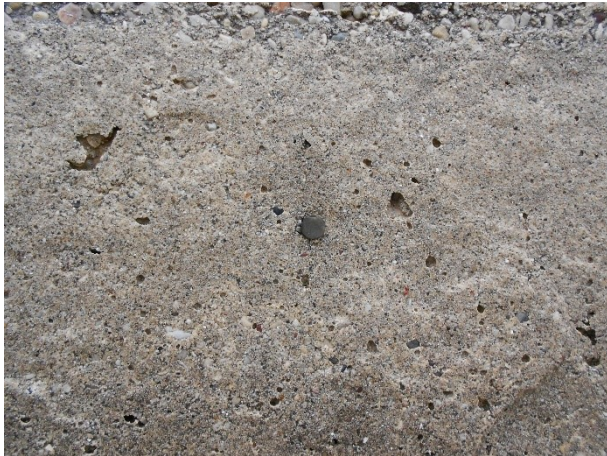
25. A close-up view of the slate texture on precast units.
