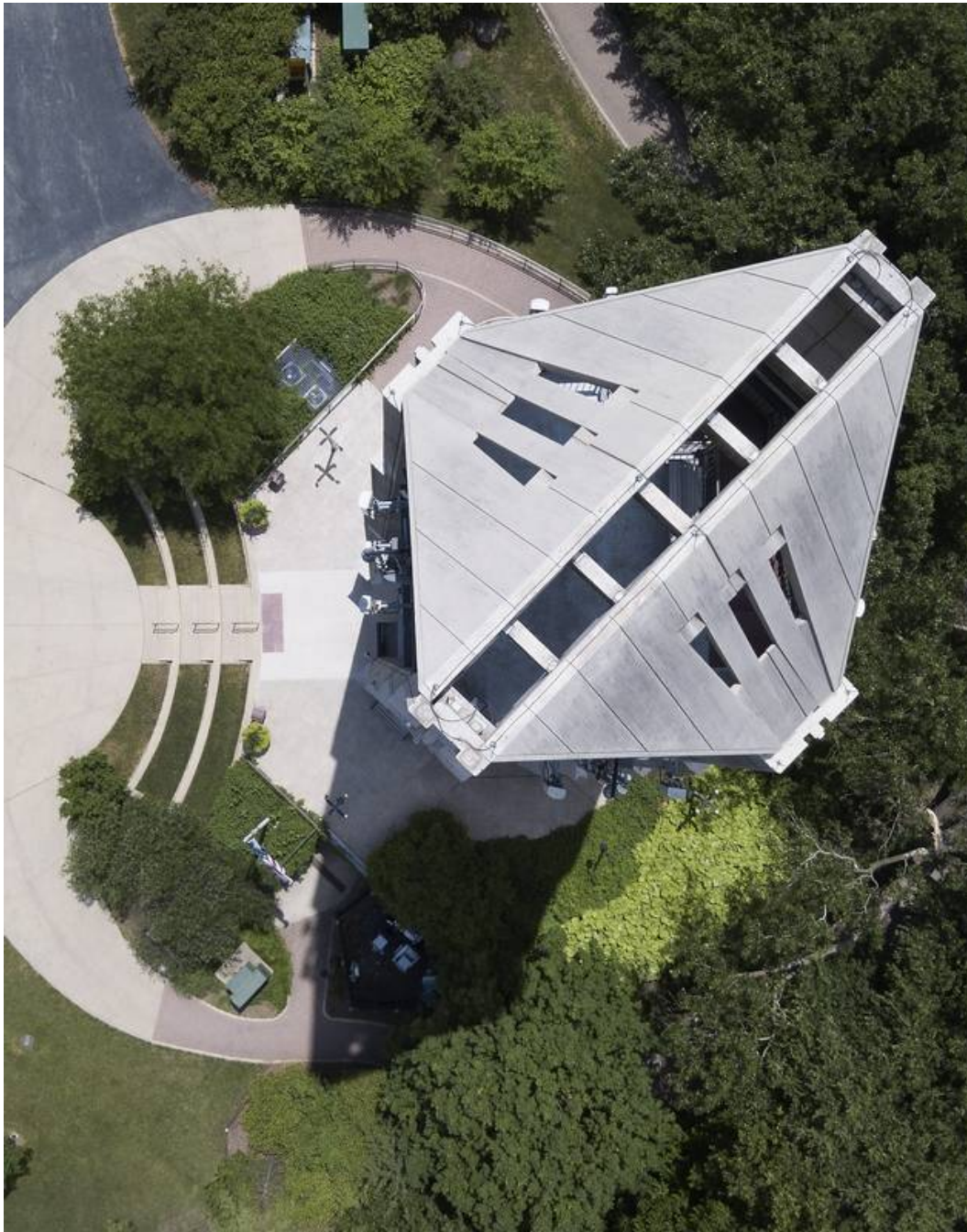
FIGURE 1 MOSER TOWER AERIAL VIEW
