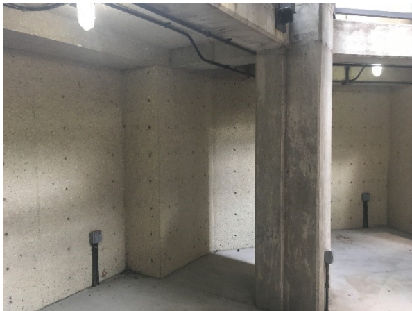
9. A view of the basement foundation walls with exposed aggregate finish.
