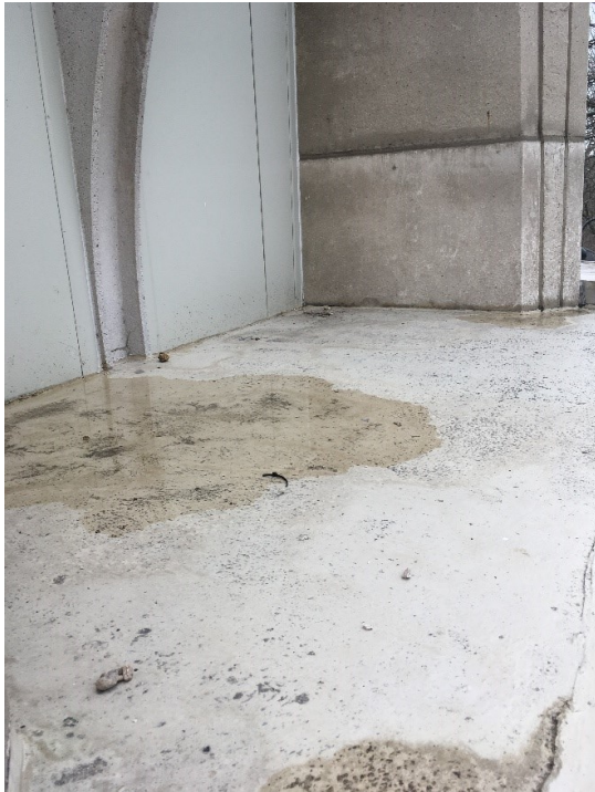
111. A close-up of the small roof at ground floor. Note standing water.
