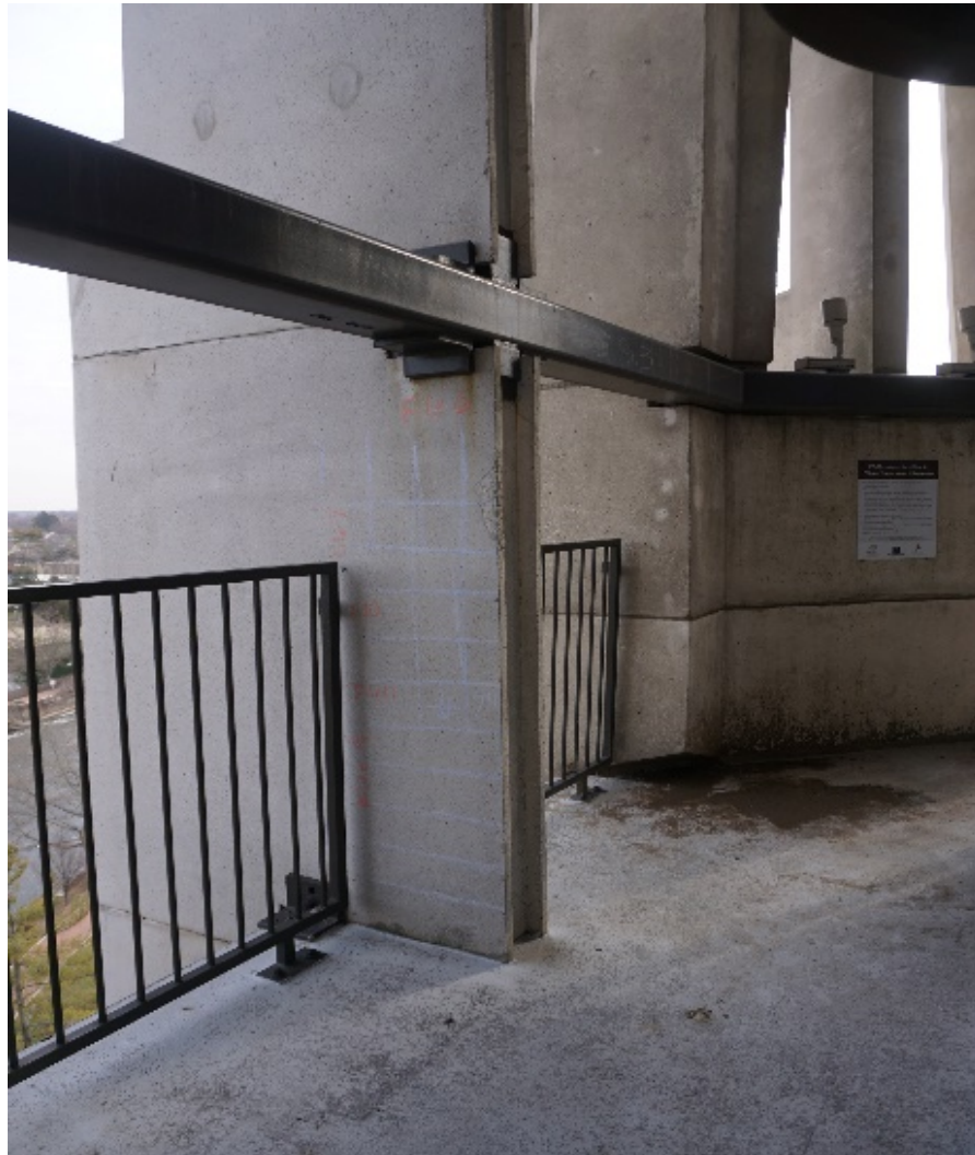
FIGURE 4 COMPRESSIVE RING AT ELEV. +81.3
