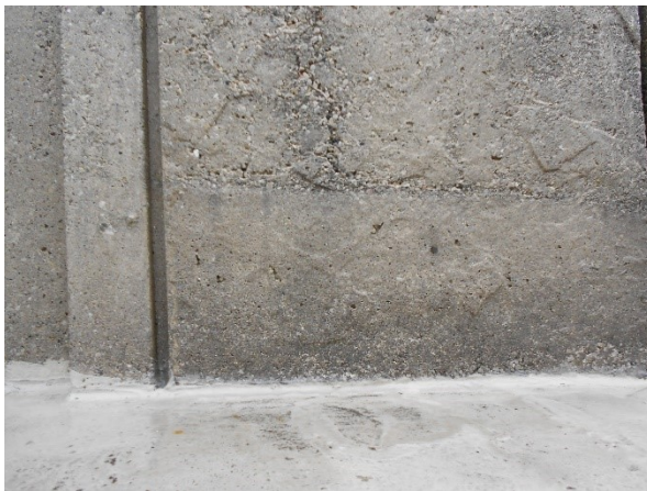
27. A close-up view of the stone textured precast units.
