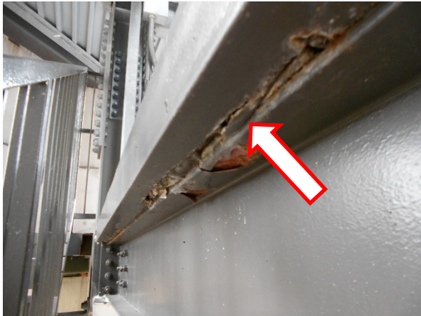
79. A close-up of corroded deck angle and Belfry level.
