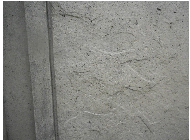
26. A close-up view of the slate texture on precast units.
