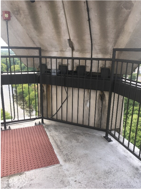
63. A view of the NW pier at the Observation deck. Note corrosion staining below the ring beam.
