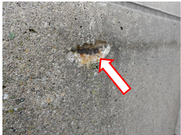
34. A close-up view of small rebar spalls
