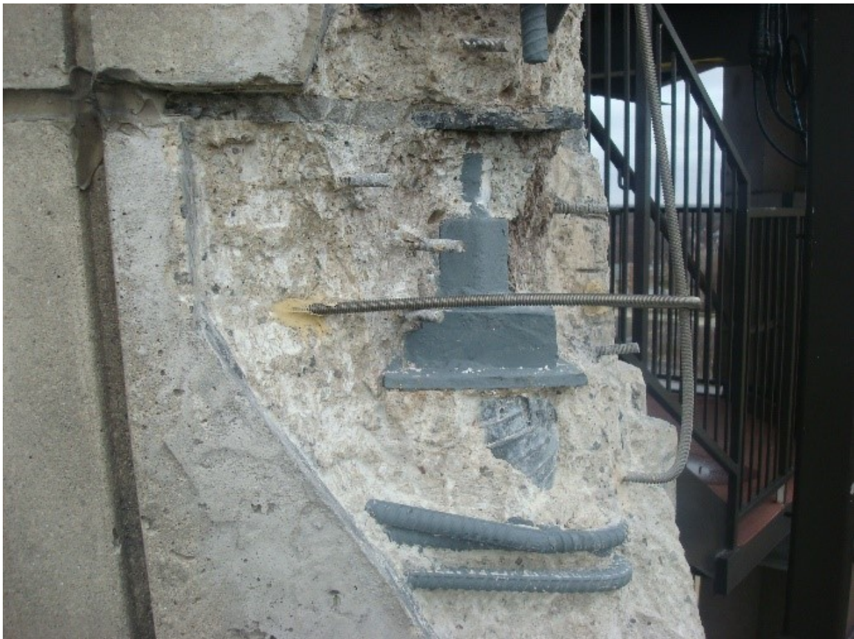
55. A close-up view of failed patch on the SE pier El.116-8" after demolition. The patch that was removed did not have sufficient anchorage to prevent a fall. The exposed concrete cast around the Dywidag post-tensioned hardware is not fully engaged with the steel. The architectural concern for this condition due to its repetition on all sides at this level is that the Dywidag is not sufficiently engaged with the structural reinforcing to prevent repeated failure.
