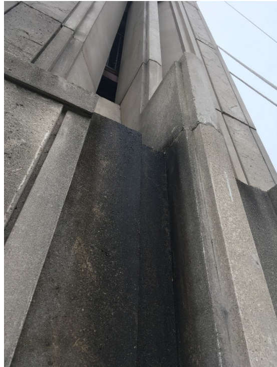
50. An example of surface discoloration from runoff.
