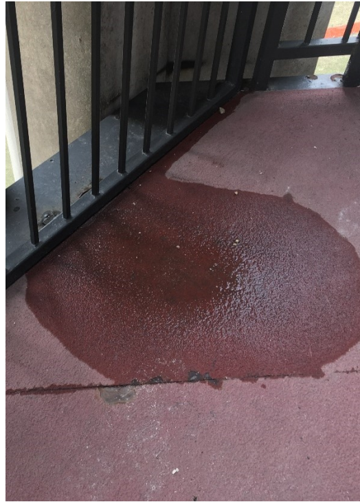
38. Standing water on stair landing.
