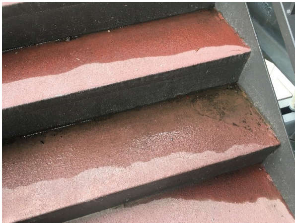
87. A close-up of steel stair with standing water and corrosion.
