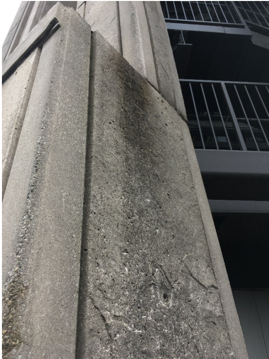
49. An example of surface discoloration from runoff.
