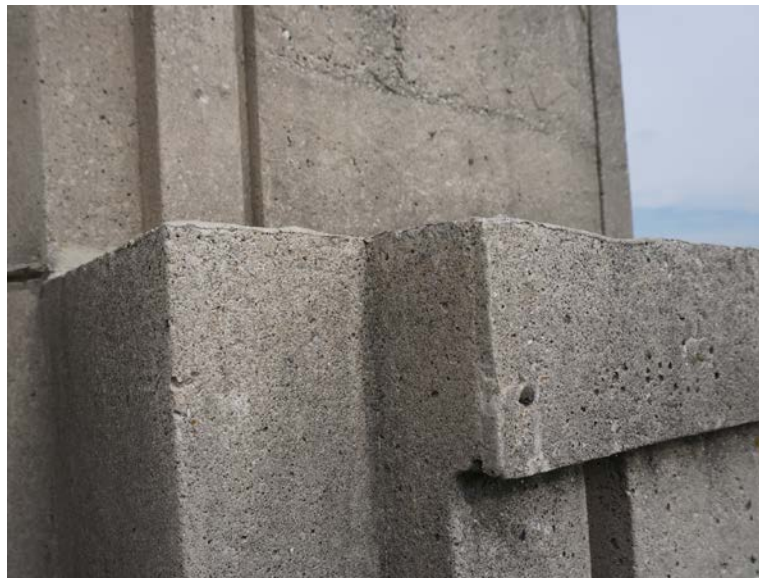
FIGURE 24 STEPPING CONFIGURATION OF THE PRE-CAST PANEL ON THE ELEVATION
