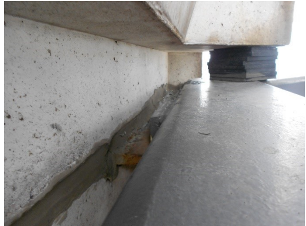
70. A close-up view of clip angle in precast concrete joint from above.
