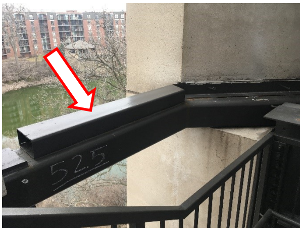
95. A view of abandoned deck support at the Gallery level.
