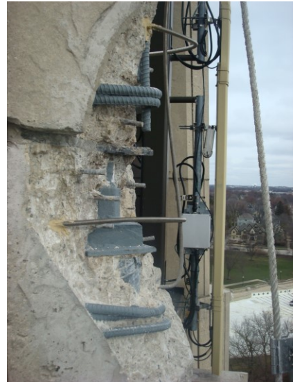
Failed patch with post-tension dead end with anchor stressing assembly. Note new stainless-steel patch reinforcing.
