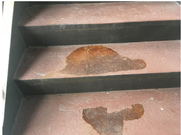
88. A close-up of steel stair with delamination of traffic coating and corrosion.
