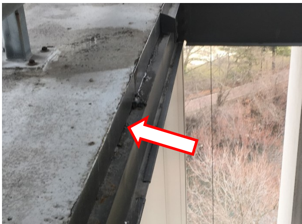
83. A close-up view of the corroded deck edge at elevator shaft at the Belfry level.
