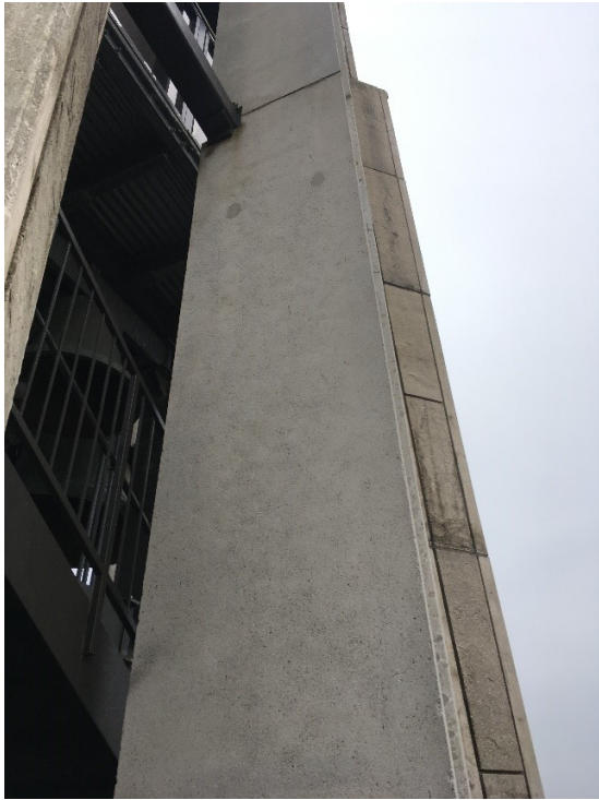
41. A view of a precast fin. Note small lift point patches.
