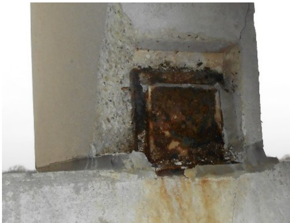
57. A close-up of failed embed patch at small precast fin in pier.
