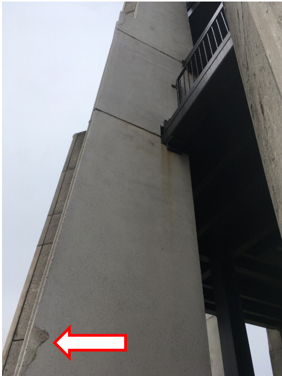
39. A view of a precast fin. Note patch at outer edge at left.
