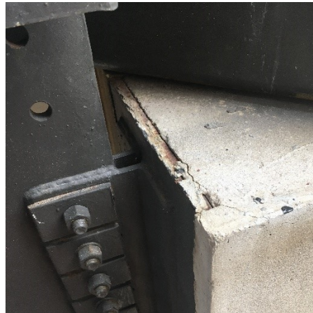
20. A close-up view of the exposed top of the steel embed at the Gallery level beam.
