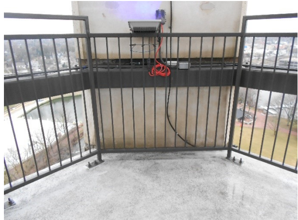
92. A view of the traffic coating on the Observation deck.
