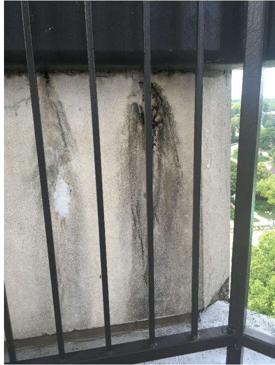
64. A close-up of corrosion and leak patterns at the NW pier below the ring beam.
