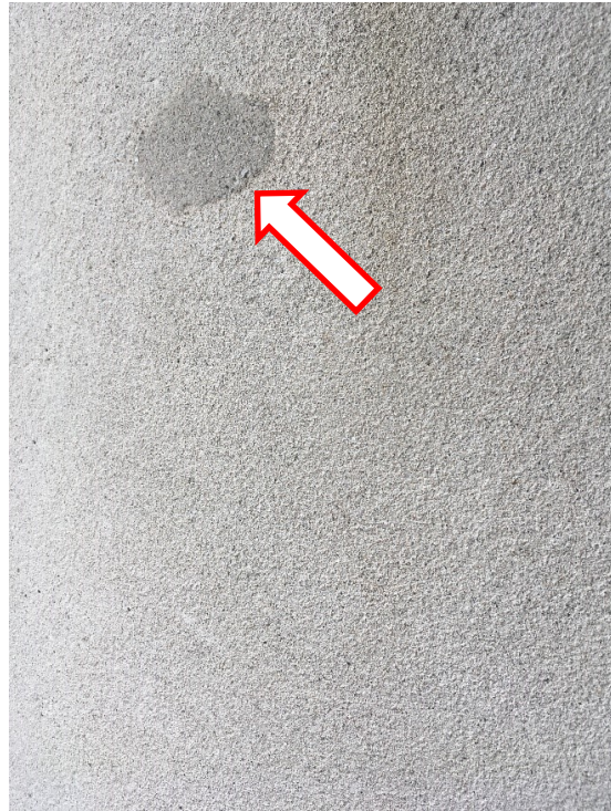
46. close-up of the precast fin showing surface finish. Note typical lift point patch.
