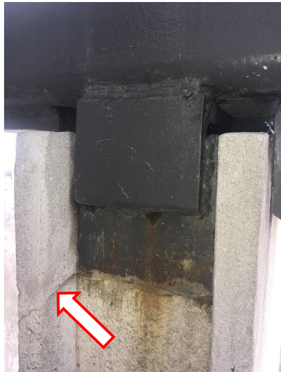
44. A close-up view of the precast fin weld connection. Note concrete crack at corner of steel embed
