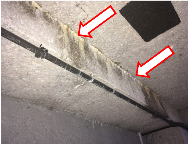
13. A close-up view of concrete cracks and water infiltration below front door.
