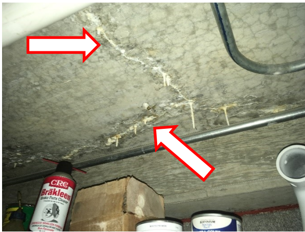
15. A view of concrete cracks and mineral leaching in mechanical room below plaza.
