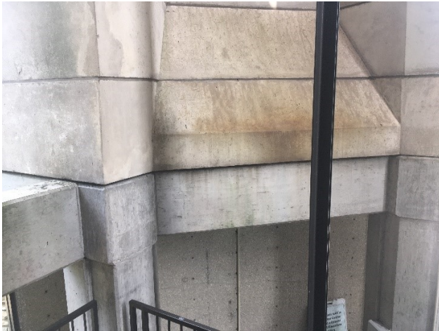
7. A view of the concrete foundation with precast unit above.
