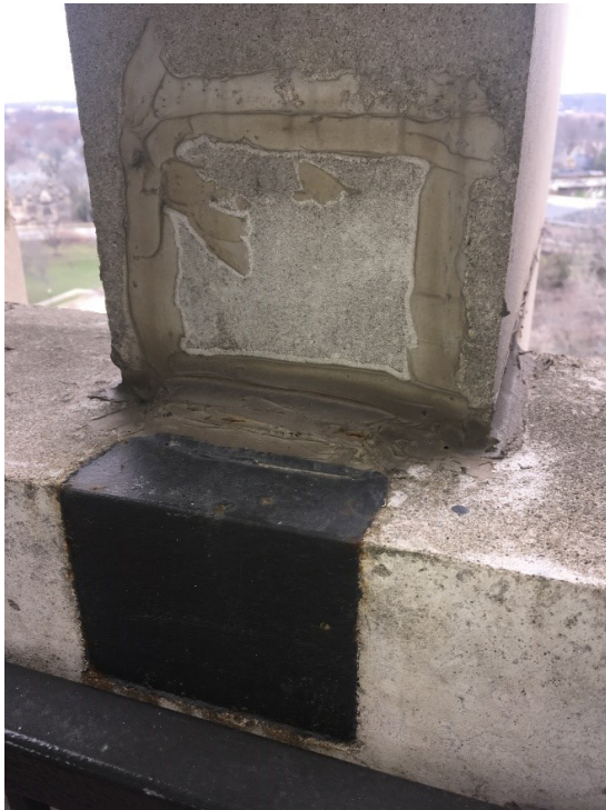
59. A close-up of an embed patch with sealant.
