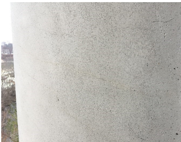
35. A close-up of a precast fin panel with several diagonal hairline cracks.
