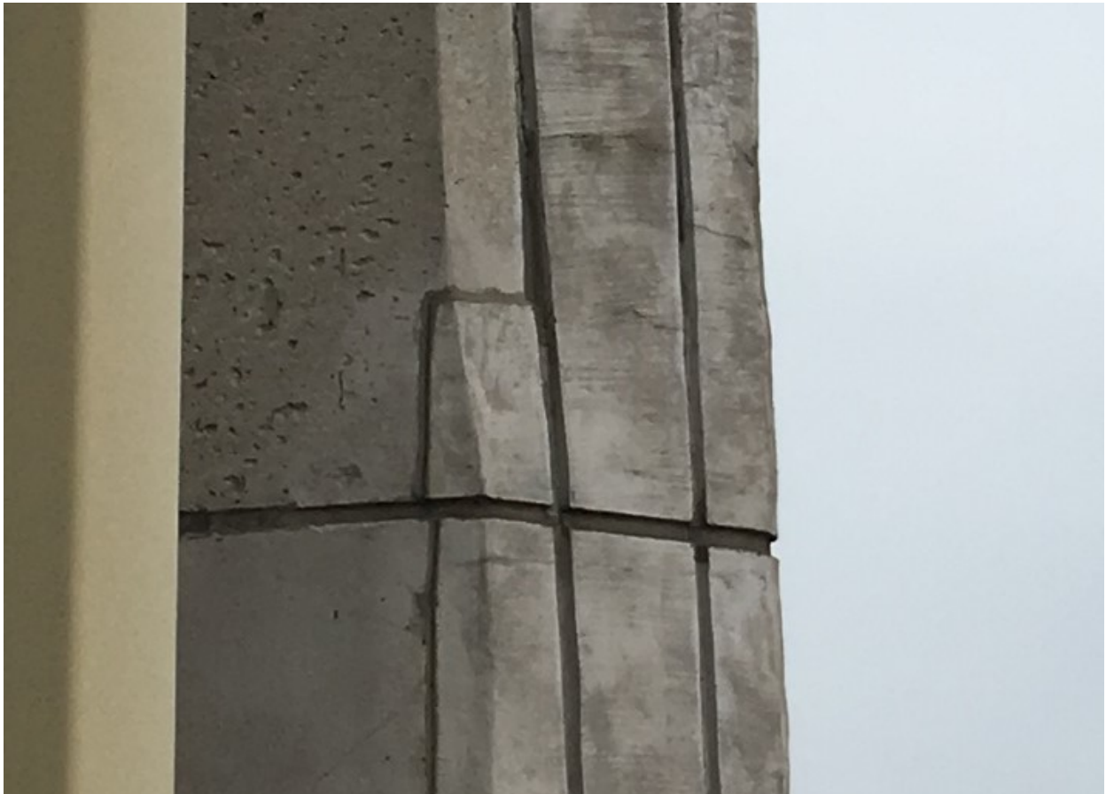
56. A view of previously made patches on the SW pier. At the same 116' elevation as photo 55. This condition is visible on all sides of the structure at this location
