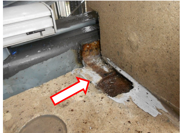
74. A view of a precast clip angle exposed at horizontal surface.
