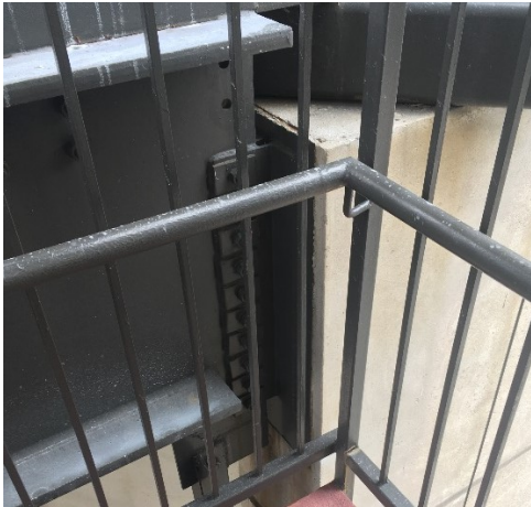
19. Wide flange beam connected to precast at the Gallery level.
