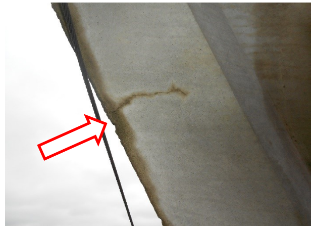
28. A close-up view of the knife edge of the roof panel with crack and water saturation.
