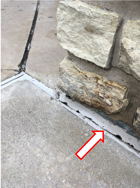
107. A close-up of the failed sealant and flashing at the stone veneer and plaza.
