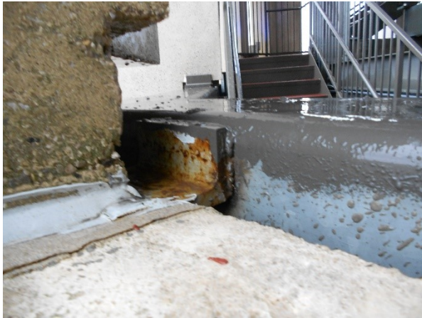
73. A view of a precast clip angle exposed at horizontal surface.
