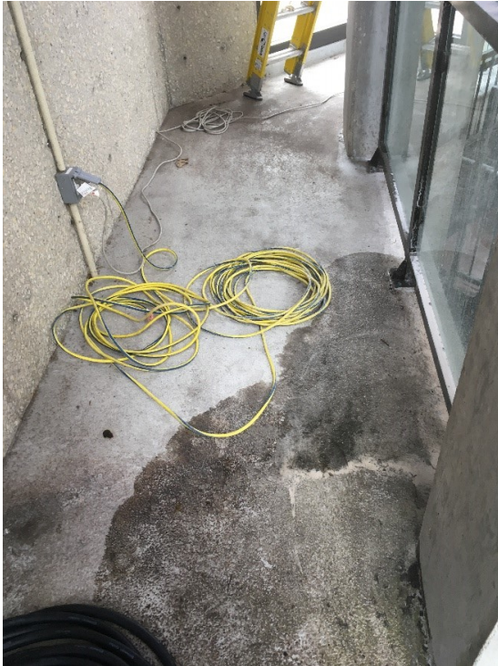
97. A view of the ground floor failed traffic coating with standing water.
