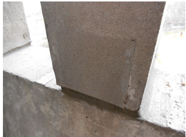
58. A close-up of an intact embed patch.
