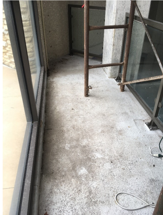
98. A view of the ground floor damaged traffic coating.
