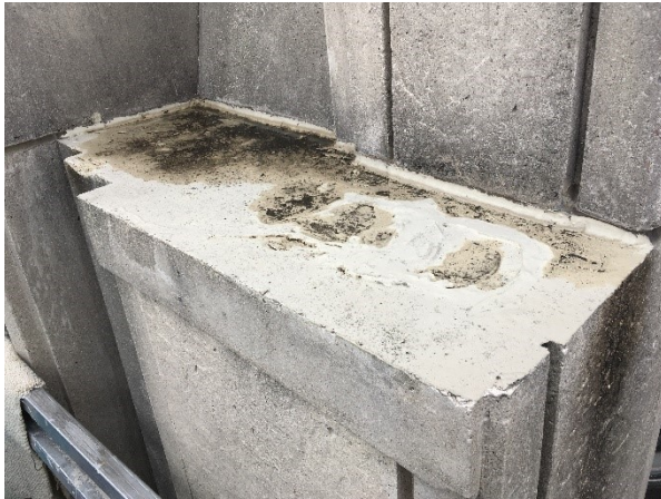
101. A close-up of precast ledge with traffic coating and standing water.
