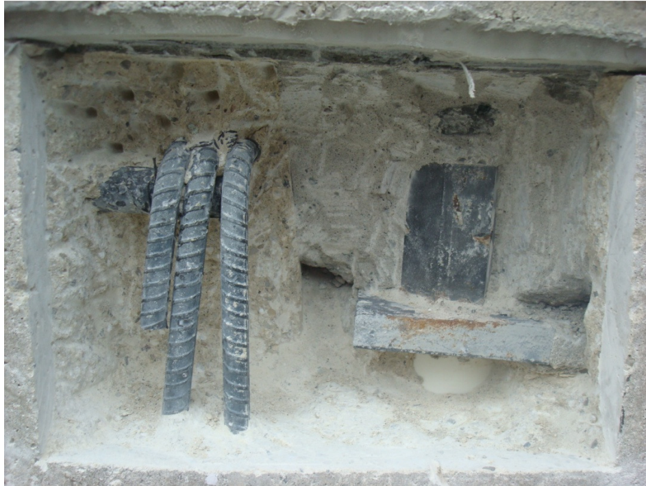
Photograph #2: Exposed end of PT rod and reinforcement bars at left opening
