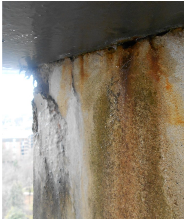
66. A close-up of corrosion and leak patterns at the NW pier below the ring beam.
