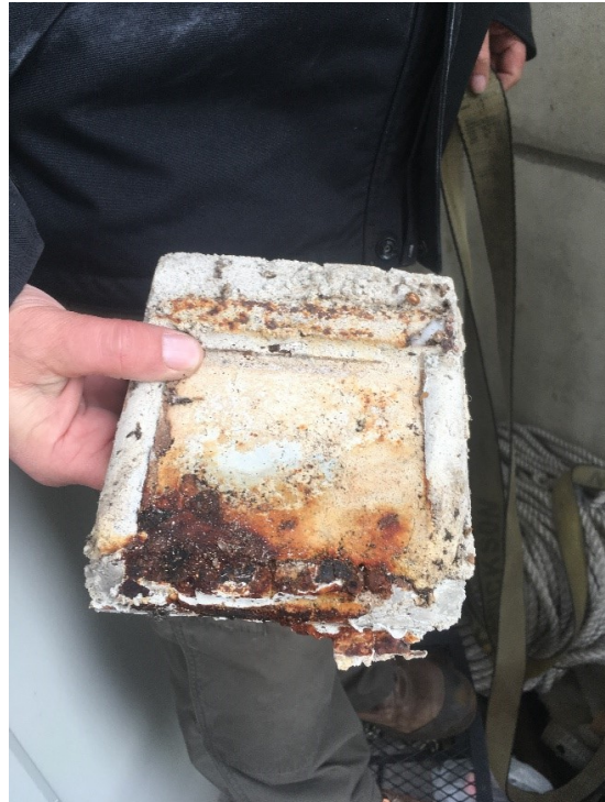
60. A failed embed patch removed during inspection.
