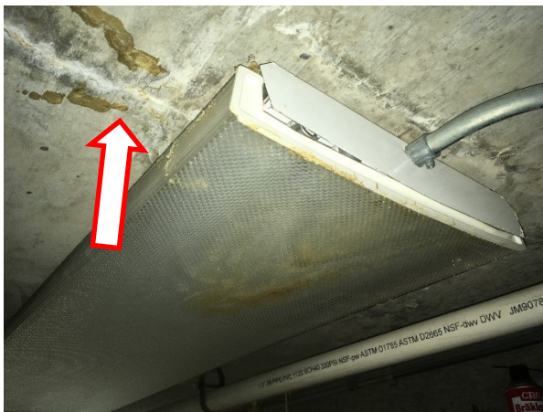
17. A view of concrete cracks and water infiltration in mechanical room below plaza.
