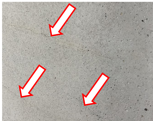
36. A close-up of precast fin panel with several diagonal hairline cracks
