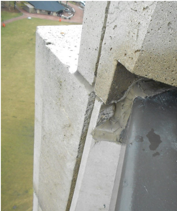
65. A close-up of ledge adjacent to the interior leaks at the Observation deck.
