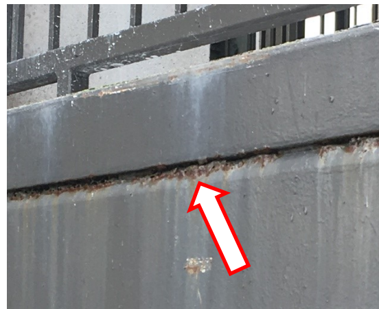
78. A view of typical corrosion at non-galvanized deck edge and ring beam.
