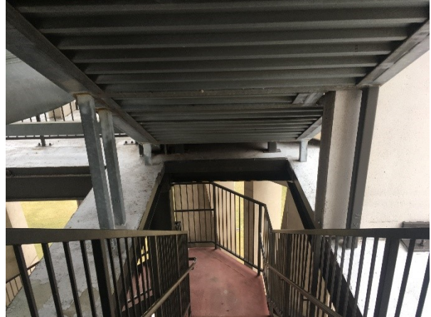
68. Galvanized roof framing at the Belfry level.
