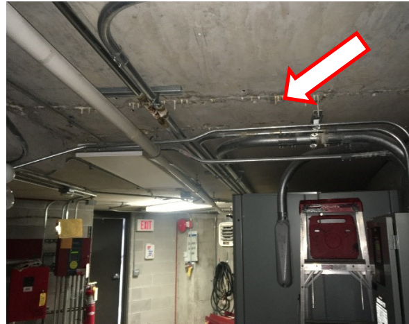
14. A view of concrete cracks and water infiltration in mechanical room below plaza.
