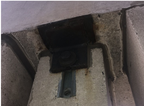
85. A close-up of fin connection in main piers.
