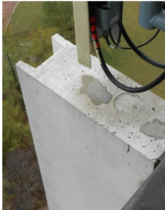
48. A view of the top of a precast fin. Note tensioning rod patches.
