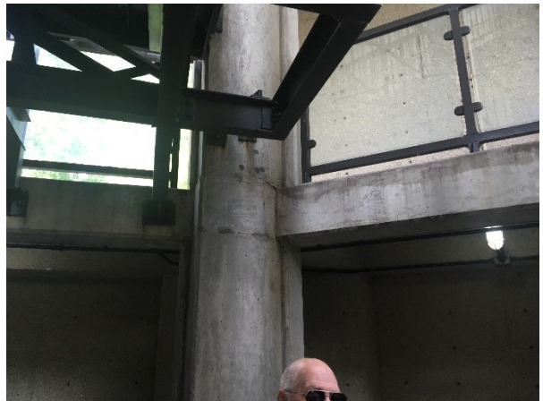
10. A view of the concrete foundation from basement level with hanging stair.
