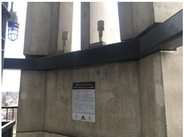
18. A view of one ring beam connection to the precast. The configuration of ring level connection varies.
