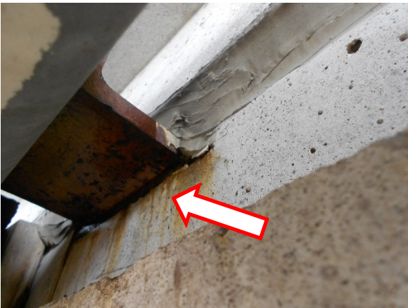
71. A close-up view of clip angle in precast concrete joint from below. Note corrosion staining from runoff.
