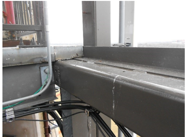
94. A view of abandoned deck support at the Gallery level.
