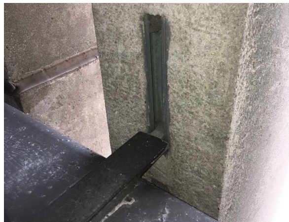
84. A close-up of fin channel embed connection in main piers.
