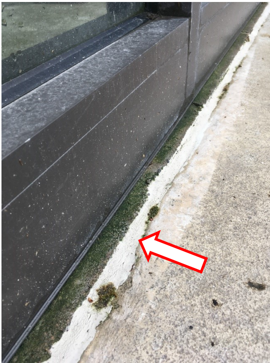
99. A close-up view of the base of glazing walls. Note failed sealant and biological growth.
