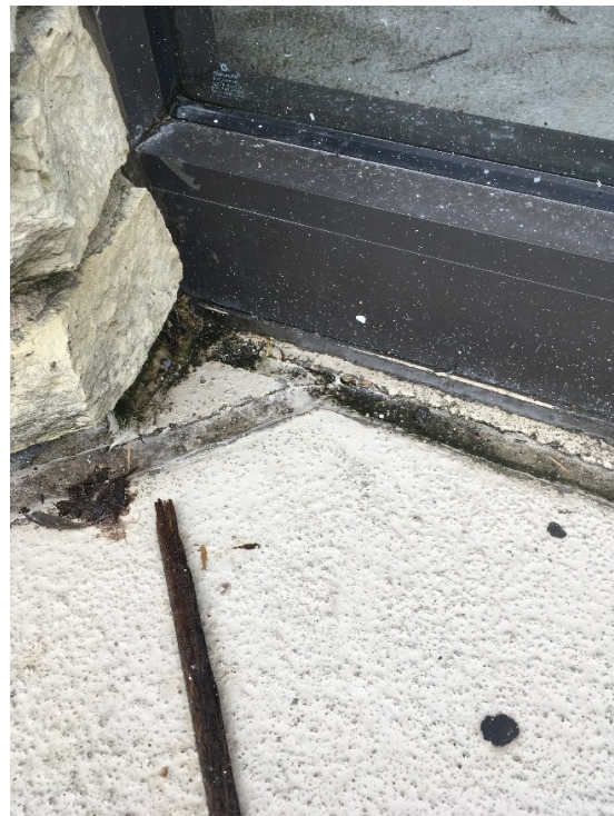
100. A close-up view of the base of glazing walls. Note failed sealant and biological growth.
