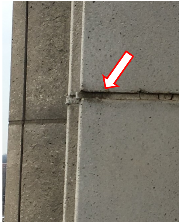
40. A close-up of view of a precast fin joint. Note loose grout in joint.
