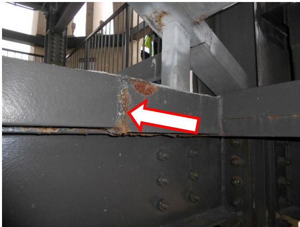
81. A close-up of corroded deck angle at the Belfry level.
