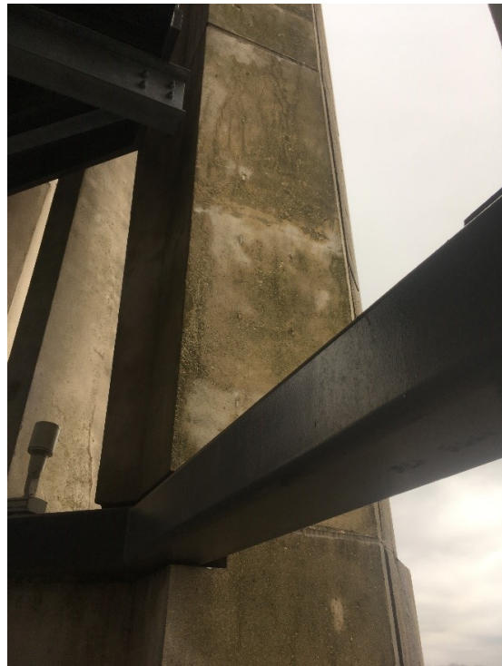
52. An example of surface discoloration from biological growth.
