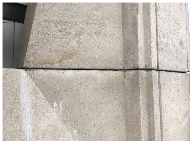
24. A view of the slate textured precast units.
