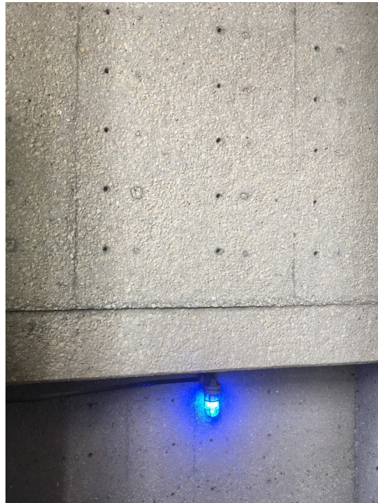
6. A detail view of the concrete foundation. Note the exposed aggregate finish.
