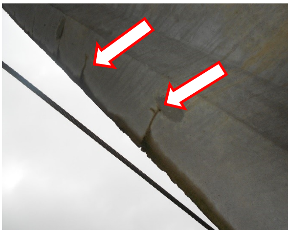
29. A close-up view of the knife edge of the roof panel with cracks and water saturation.
