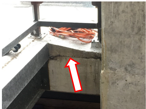
96. A view of the edge of the sloped topping slab at the ground floor.
