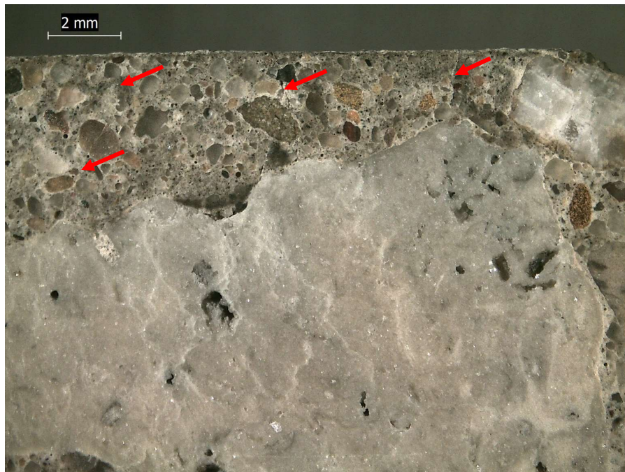
Figure 29. Column (3150054). Stereo-optical micrograph of the polished slab showing perpendicular microcracks consistent with drying shrinkage up to 3/16" deep.
