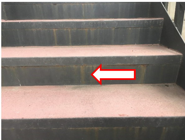
89. A close-up of steel stair with corrosion runoff stains from uncoated metal to metal contact.
