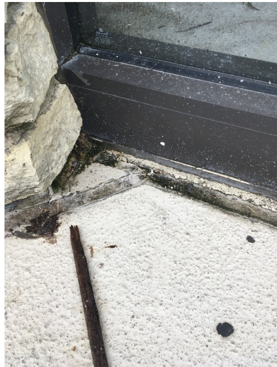
110. A close-up of the failed sealant and flashing at the stone veneer and plaza.
