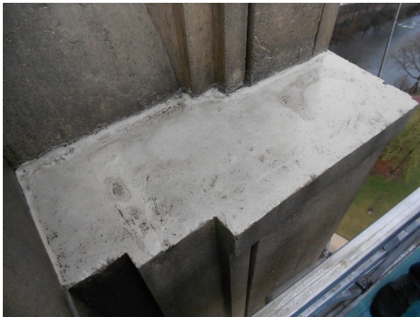
103. A close-up of precast ledge with intact traffic coating.
