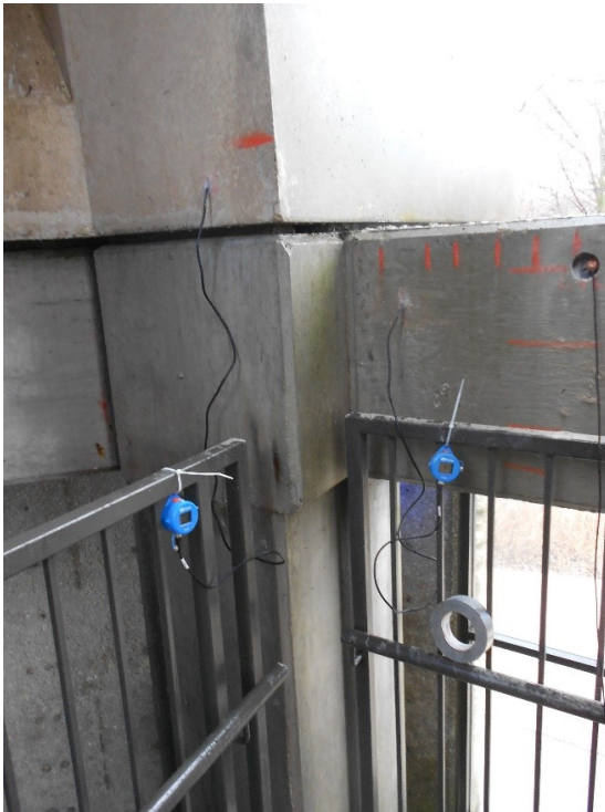
5. A detail view of the concrete column and beam with precast unit above.
