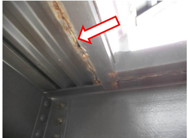
80. A close-up of corroded deck angle and Belfry level.
