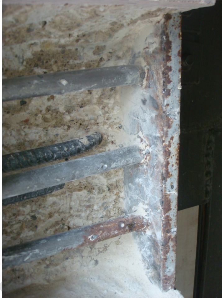
Photograph #6: Backside of connection plate and embedded studs at northeast side of Elev. 52.5.
