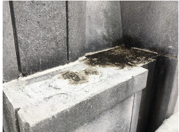
102. A close-up of precast ledge with traffic coating and standing water.
