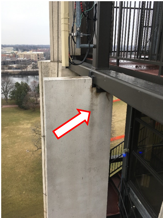
47. A view of the top of a precast fin. Note corrosion and runoff stains.
