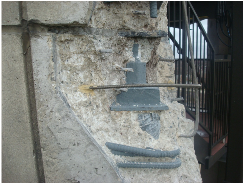
Photograph #4: Exposed end of PT rod and reinforcement bars at right opening
