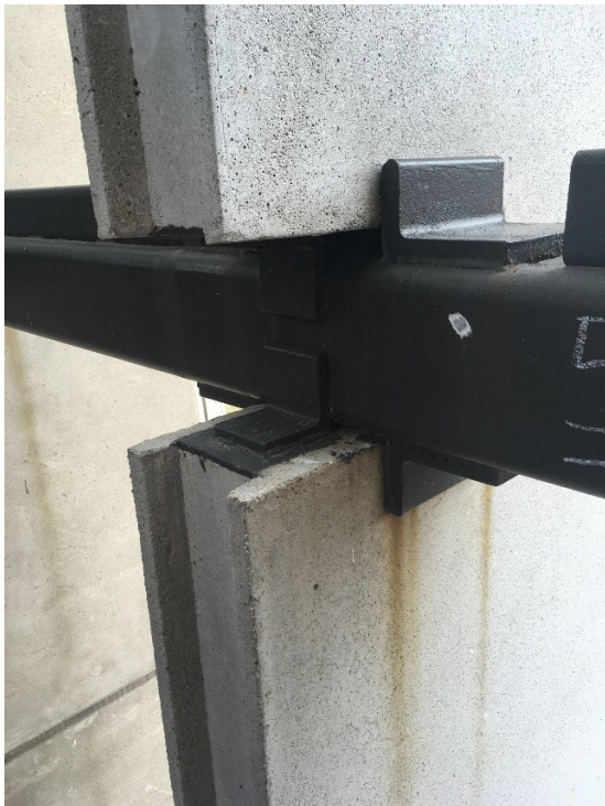
43. A detail view of the precast fin connection. Note corrosion staining.
