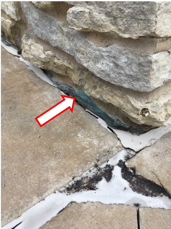
109. A close-up of the failed sealant and damaged flashing at the stone veneer and plaza.
