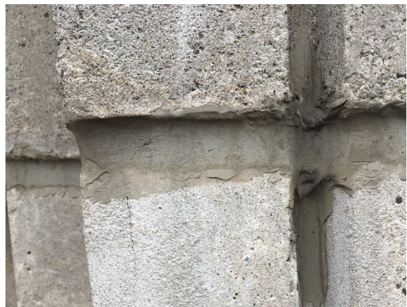
106. A close-up of typical precast sealant joint.
