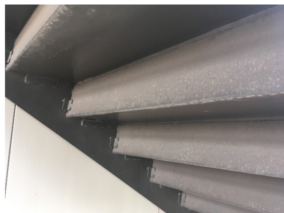
90. A close-up of bottom of steel stair with supporting clip angles.
