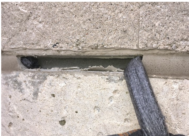
105. A close-up of 1 of 2 sealant probes performed during the investigation.
