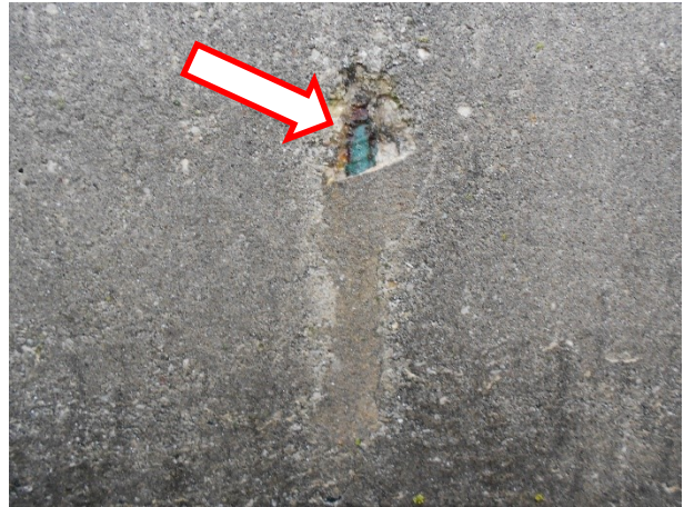
32. A close-up view of a small rebar spall. Note the previous patch.
