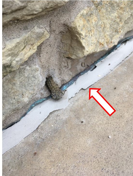
108. A close-up of the failed sealant and damaged flashing at the stone veneer and plaza.
