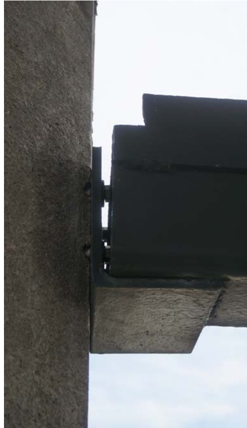
FIGURE 23 DETAIL OF CONNECTION BETWEEN COMPRESSIVE RING AND THE PRE-CAST PANEL
