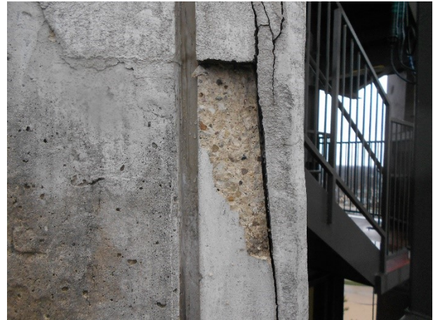
54. A close-up view of failed patch at El. 116'-8" prior to repatching. .
