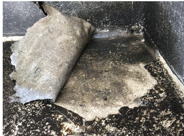
104. A close-up of precast ledge with failed waterproofing and standing water.
