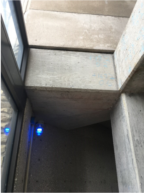
3. A detail view of the concrete foundation with precast unit above.
