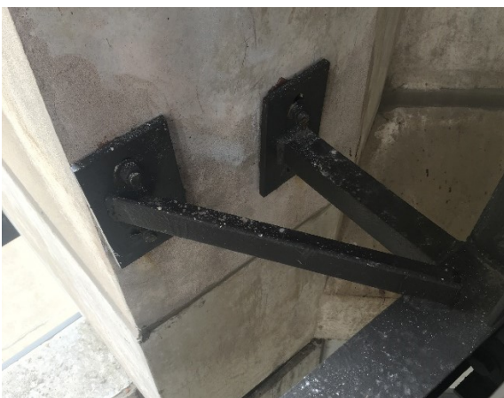
23. A view of the lateral braces for the hanging stair structure attached to channel embeds.
