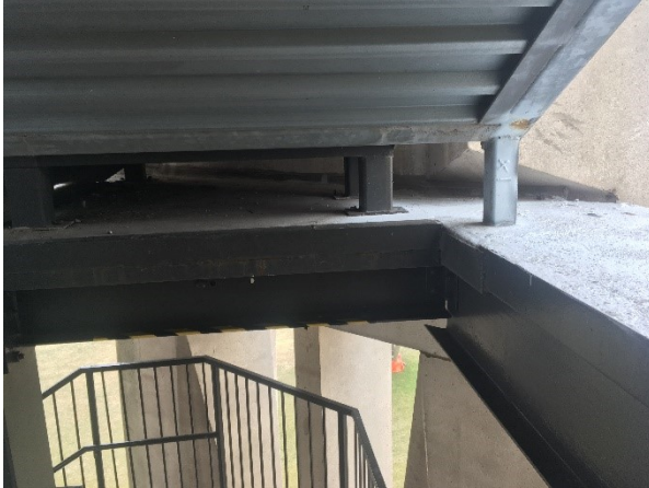
67. Galvanized roof framing at the Belfry level.
