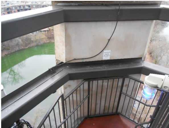
93. A view of abandoned deck support at the Gallery level.
