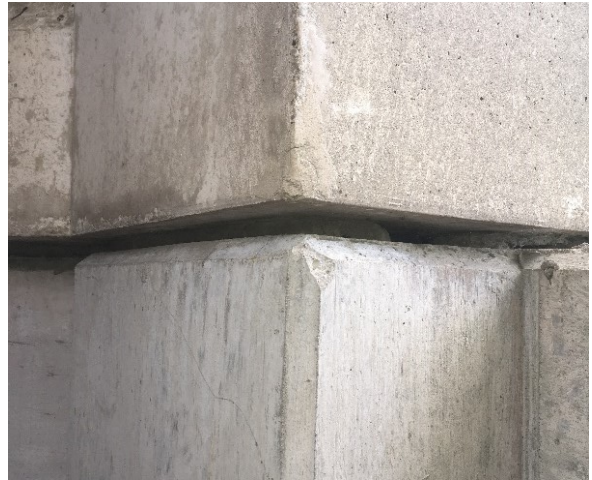
8. A close-up view of the concrete foundation with precast unit above.
