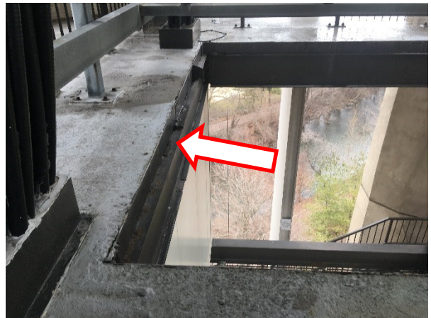
82. A view of the corroded deck edge at elevator shaft at the Belfry level.
