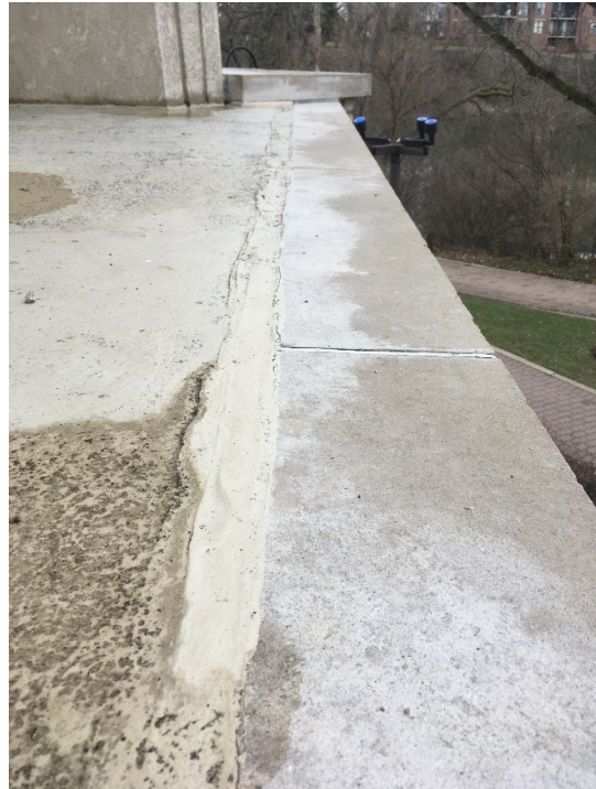
112. A close-up of the failed sealant at the West side of ground floor coping.
