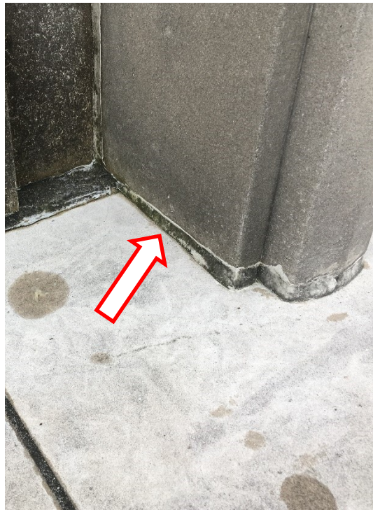
114. A close-up of a precast fin intersecting the Northwest base coping. Note failed sealant.
