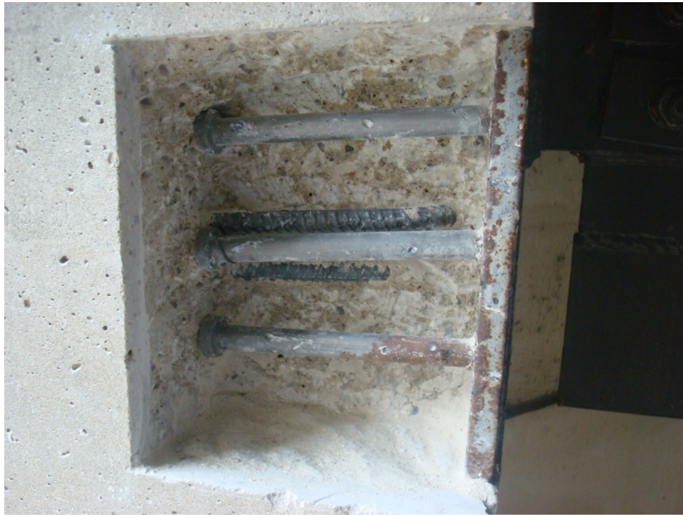
Photograph #5: Exposed connection plate and embedded studs at northeast side of Elev. 52.5.
