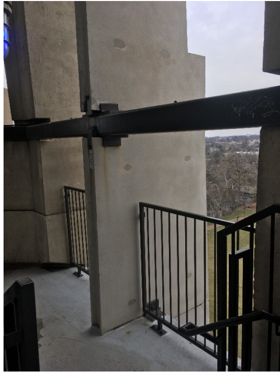
42. A view of a precast fin connection. Note small lift point patches.
