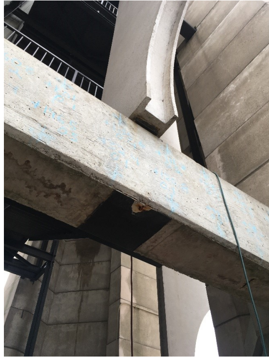
4. A detail view of the concrete beam supporting precast fin above.
