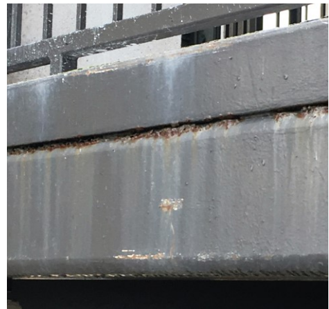
The typical corrosion buildup between ring beam and deck edge. Note vertical streaks from water runoff.
