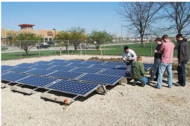
Solar panel installation
