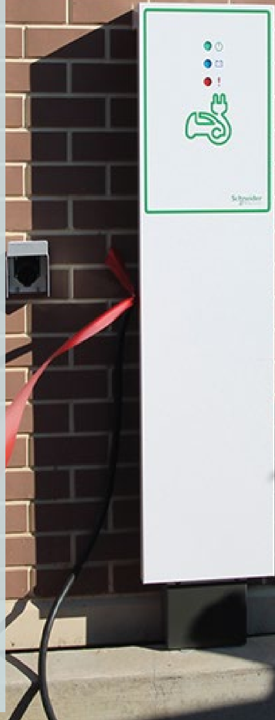
The City installed its first public Electric Vehicle Charging Station (EVCS) in the VanBuren Public Parking lot in downtown Naperville.
