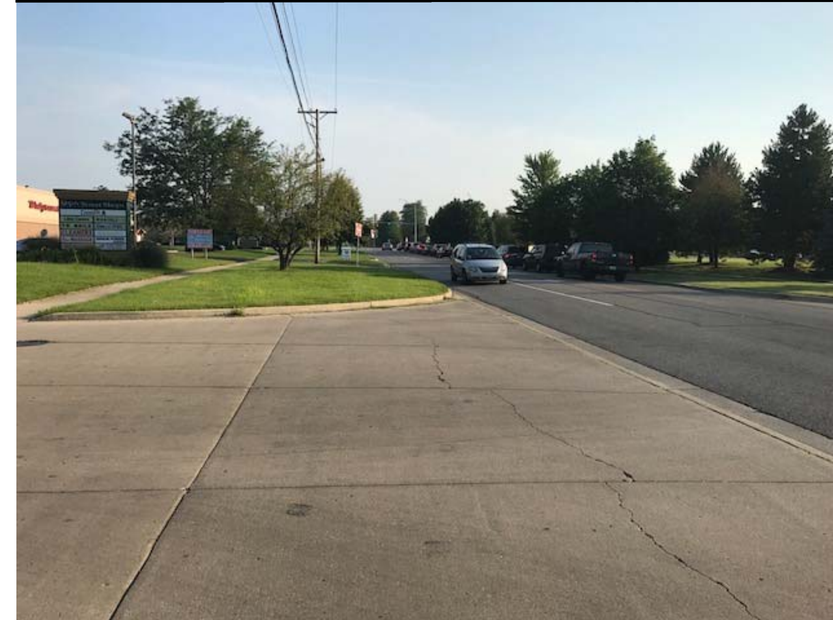
At Commercial Entrance, West Leg, Looking North along Book Road
