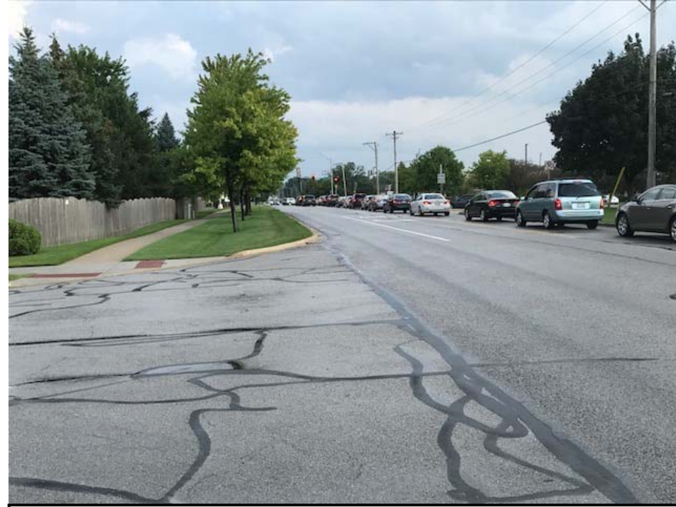
At Tamahawk Lane, East Leg, Looking South along Book Road
