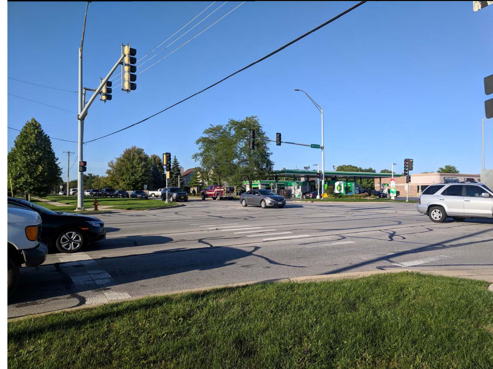
At Southwest Corner of Intersection, Looking Northeast along Book Road
