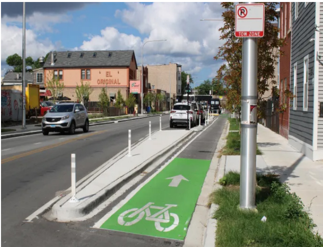
Image 16: Curb-Protected Bike Lane, Chicago, IL Source: Quinn Myers, Block Club Chicago
