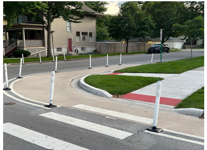
Image 31: Paint & Post Bump-Out, Oak Park, IL
