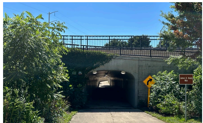
Image 27: DuPage River Trail Underpass, Naperville, IL
