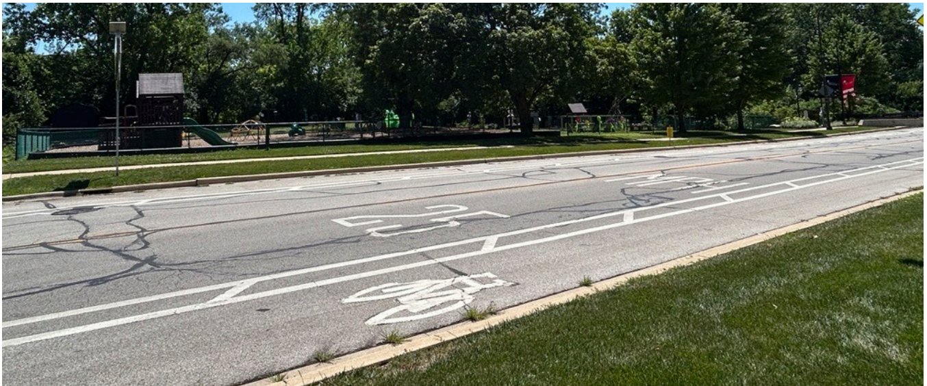
Image 24: Buffered Bike Lane, Naperville, IL
