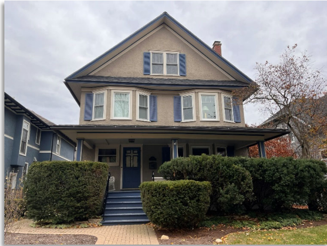
In-Kind Window Replacement, 146 N. Columbia Street
