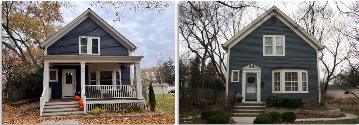
Historically Appropriate Porch Addition, 24 S. Columbia (2007 condition at right, 2025 condition at left)
