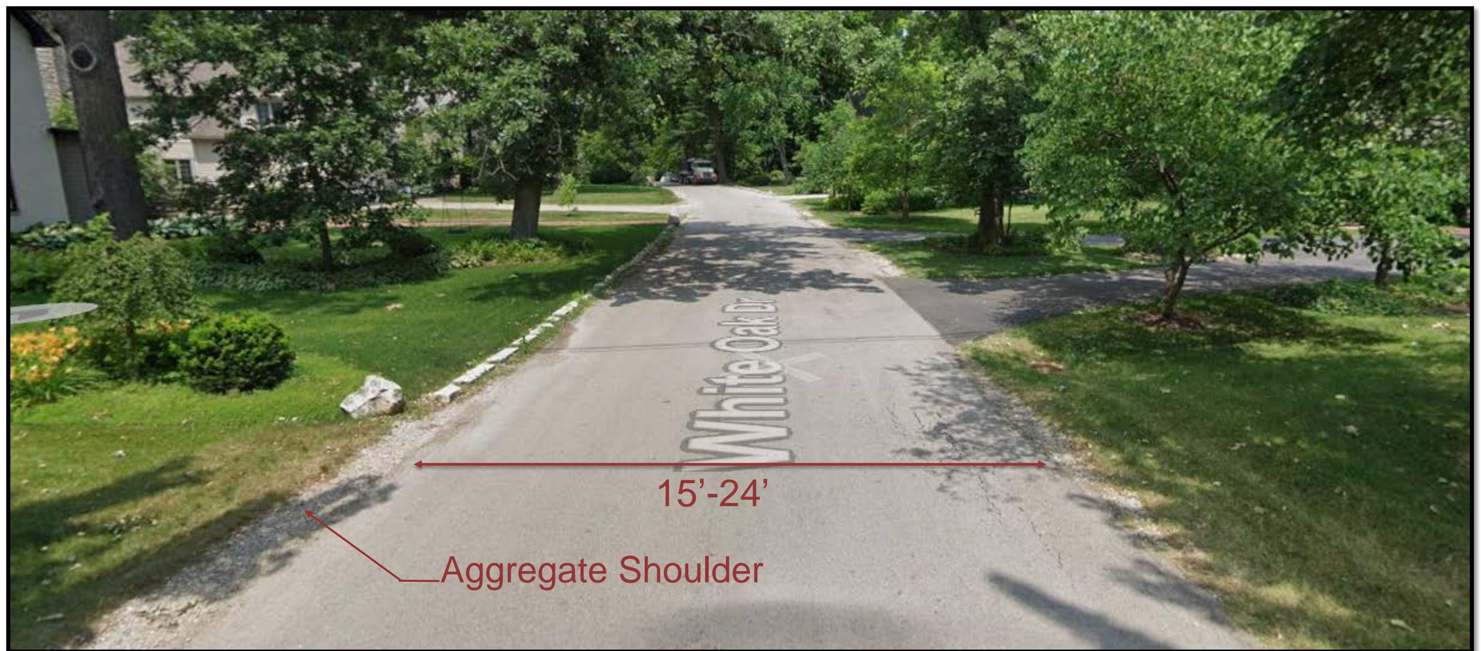
The existing pavement in the project area varies between 15' and 24' wide with variable width aggregate shoulders from 1.5' to 4'
