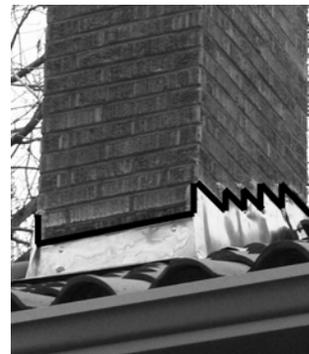
*Photo D.8 - Step flashing where chimney meets roof*
