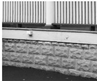
Photo D.5 - Stamped concrete - rock face finish foundation wall example
