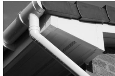
Photo D.25 - *Discouraged* - PVC gutter and downspout with metal soffit
