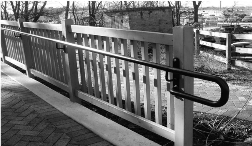
Photo E.4 - *Acceptable* - Wood baluster style ramp with customized lumber
