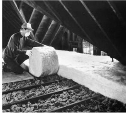
Photo D.43 - Installation of insulation blanket over sprayed cellulose insulation
