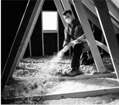
Photo D.42 - Installation of sprayed cellulose insulation
